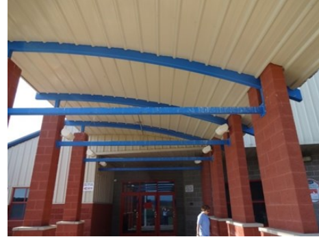
Crossbars supporting a walkway canopy are an ideal place for birds to roost. Photo: UT EPP
