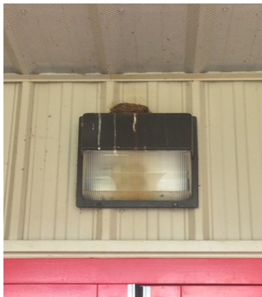
Light fixtures with flat tops invite birds to build nests. Photo: UT EPP
