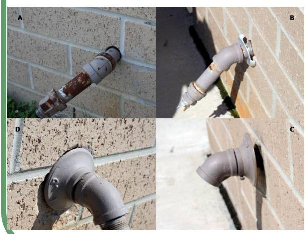
How not to install an outdoor escutcheon plate. A. Outdoor pipe penetration lacking an escutcheon plate, B. Outdoor broken escutcheon plate. C. Outdoor escutcheon plate not sealed to wall. D. Escutcheon plate pressed to wall, but not sealed around edges. Photo credit: UT E&PP, J. Maples.
