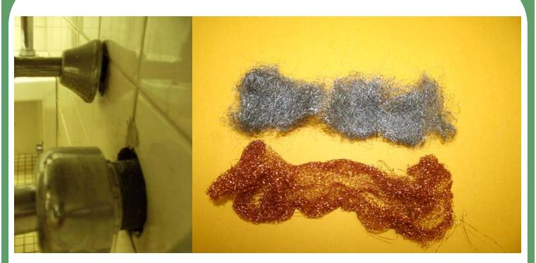
Two unsealed indoor escutcheon plates in one shot! Photo credit: UT E&PP, K. Vail. Steel wool (top) and copper mesh (bottom) can be used to fill small holes where air flow is needed. Steel wool can rust and thus degrade, and stain surfaces, so copper mesh is often preferred. Photo credit: UT E&PP, J. Maples.
