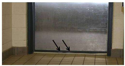
Door in a need of sweep. Light can be seen under the door indicating the door is sealed poorly. Photo credit: UT E&PP, J. Maples.
