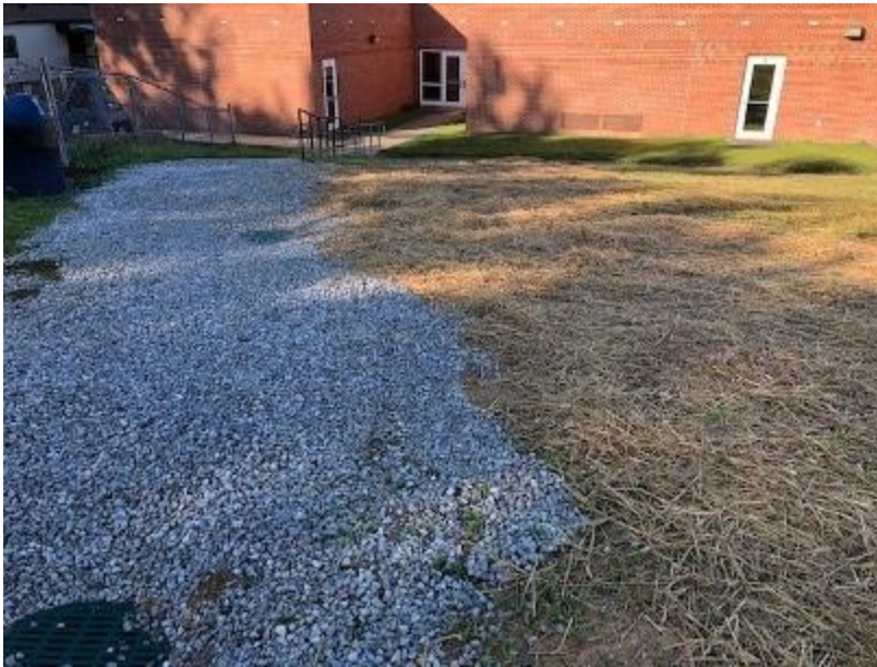
Rock covers the drainage system and fills the deep rut that had developed during previous storms.
