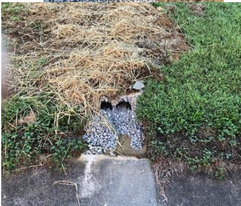
Drain pipes empty into concrete drainage channel near base of school.
