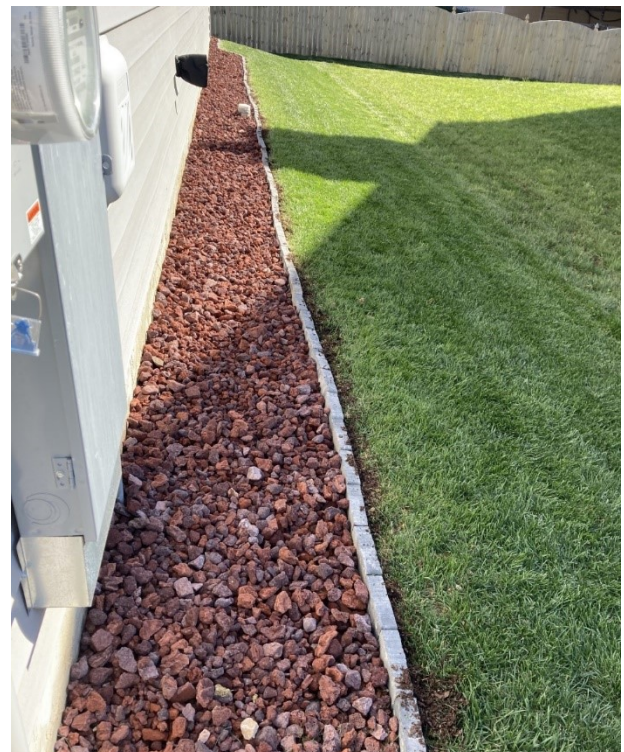
Figure 4. Placing rock or other inorganic mulch next to the foundation base should reduce the risk of clover mites wandering indoors. Credit: email submission.
