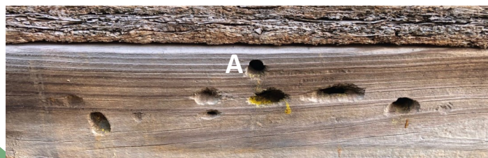
Carpenter bee gallery openings are typically 1/2 inch in diameter and round (A). The other elongated openings are probably due to woodpeckers enlarging the hole to find their prey. Credit: K. Vail, UT EPP
