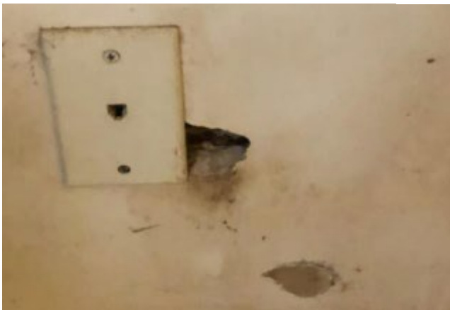
Figure 9. House mice entry point beside a faceplate. Note oily rub mark at the hole entrance. Photo: Susannah Reese, Stop-Pests.org.
