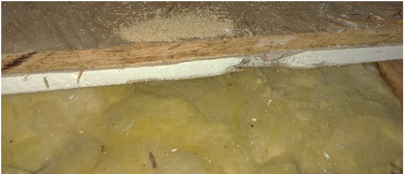
Figure 8. Western drywood termite, Incisitermes minor , alates were flying when we opened the hatch to an East Tennessee attic. Significant damage and piled termite fecal pellets were found on the floor joists throughout the attic of a decades old infestation. Credit: Karen Vail, UT E&PP
