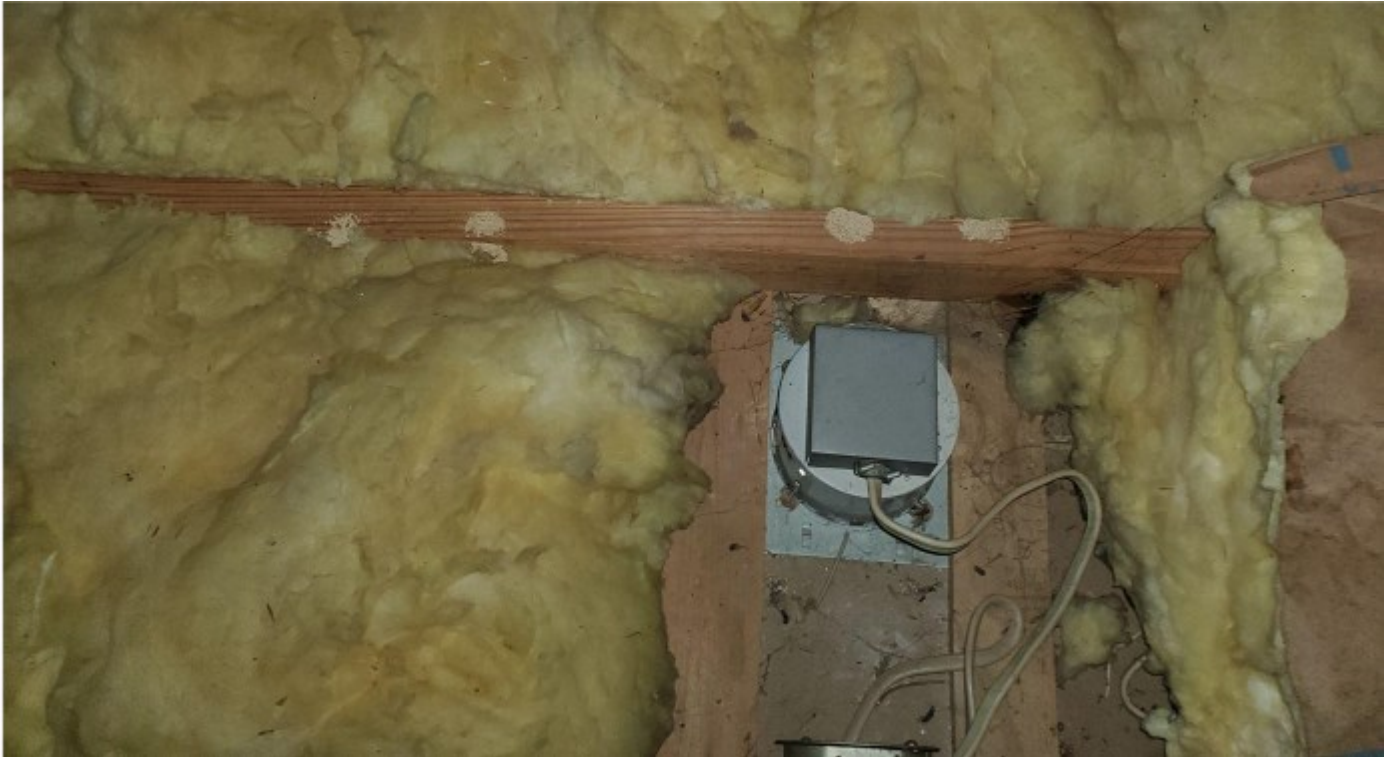
Figure 9. Drywood termite fecal pellets piled on the attic floor joists. Normally, the fecal pellets fall to the ground, but the insulation on the sides of the board prevented the termites from creating a side gallery opening. Credit: John Cook, Massey Services
