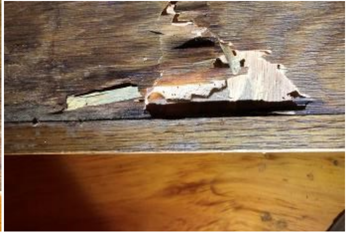
Figure 4. Above left, drywood termites leave a thin layer of wood for protection, but the thin wood may pucker. Above right, a drywood termite chamber with a few fecal pellets revealed below the puckering. Credit: Karen Vail, UT E&PP
